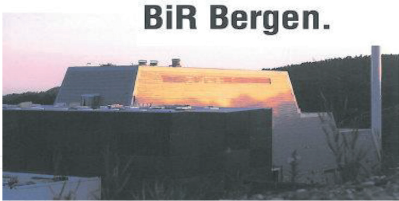
Figure 5. BiR Bergen incineration facility of 90,000 tons/year of waste with energy output about 60 GWh. Waste return in form of electricity and heat [17].
