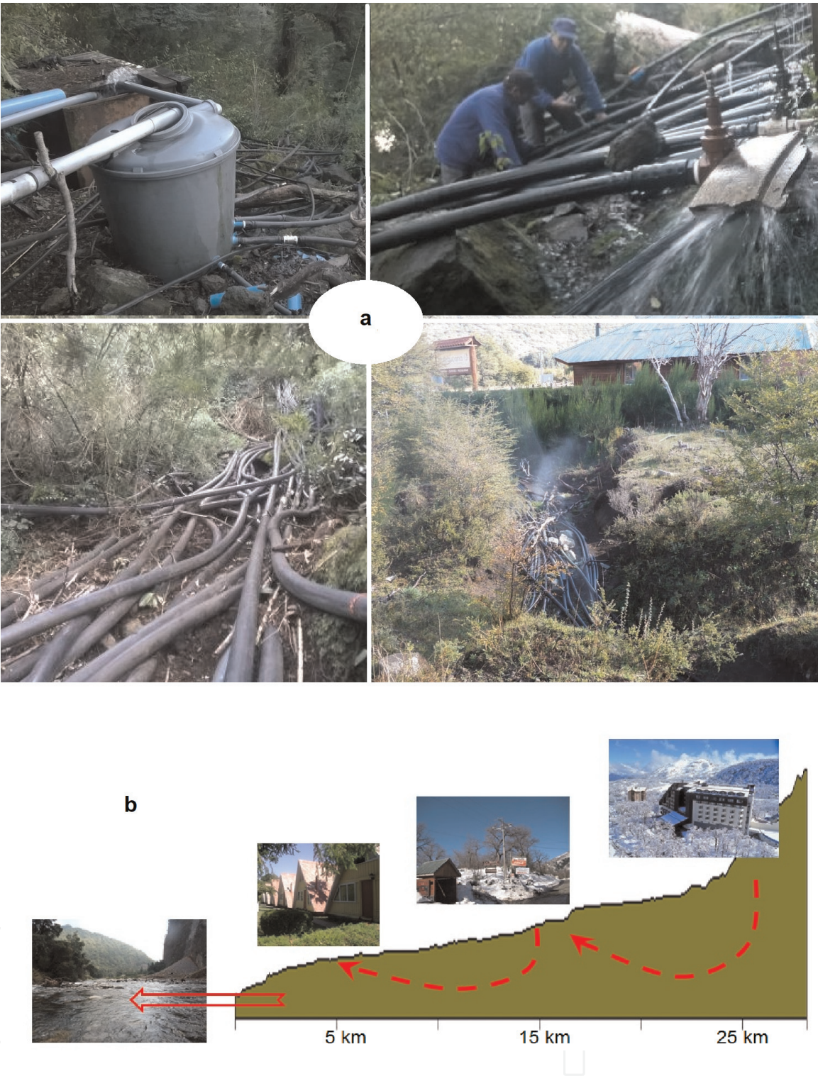
Figure 8. (a) Chaotic drinking water distribution system at the Renegado Valley; (b) scheme of the plausible pollutants' recharge and discharge processes along the Renegado Valley.
