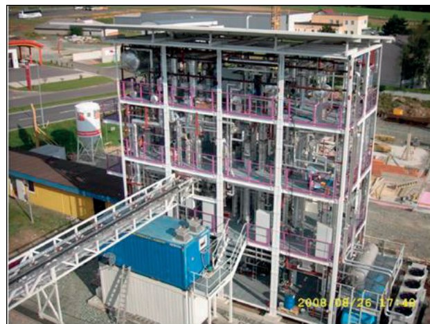
Figure 4. 1 MW capacity SNG demonstration plant [43].
