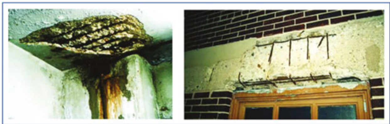
Figure 2. Deterioration of normal concrete [7].
