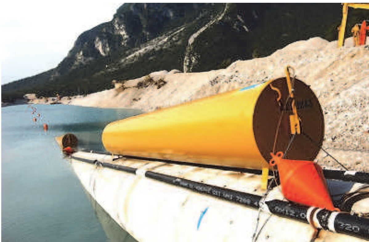
Fig. 2. Launch of a submerged methan pipe. The buoys along the launched lenght are in full view.
