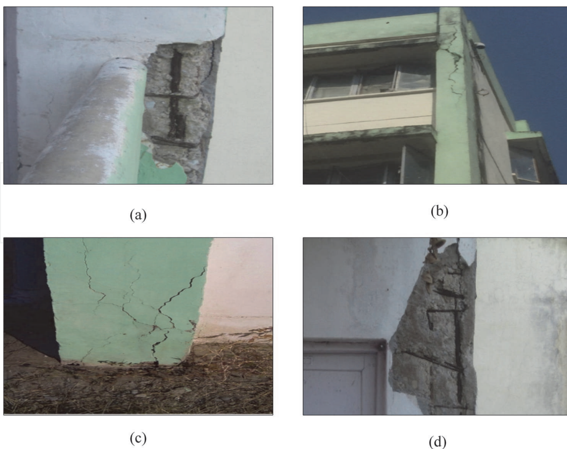
Figure 3. Damage detection (a) spalling of concrete, (b) vertical cracks on column surface, (c) cracks in the bottom of column, (d) corrosion in steel.
