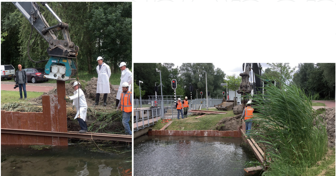
Figure 11. Installation of retaining wall by vibrating profiles with EoL composite in the soil [3].
