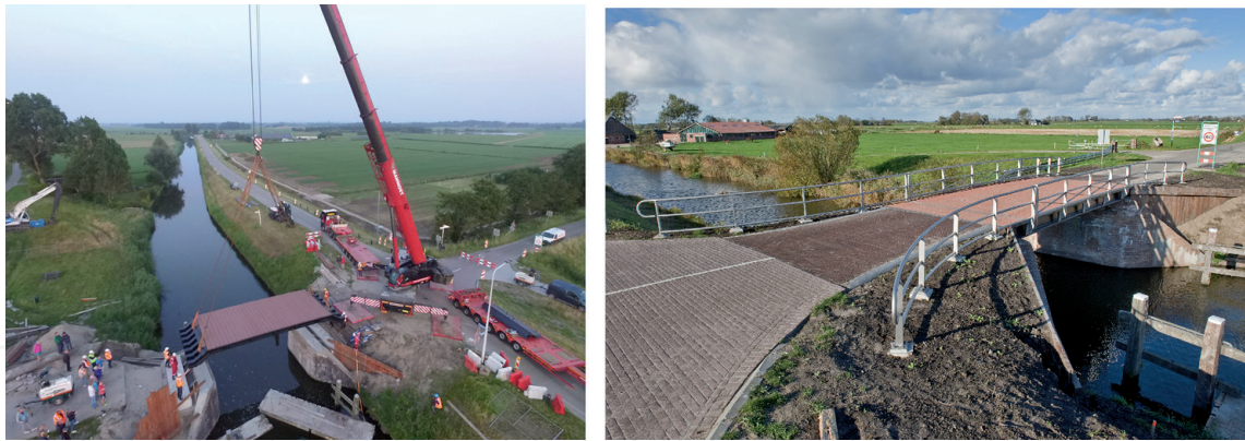
Figure 15. Dinzer bridge with deck profiles of re-used composite: Installation and final result [15].
