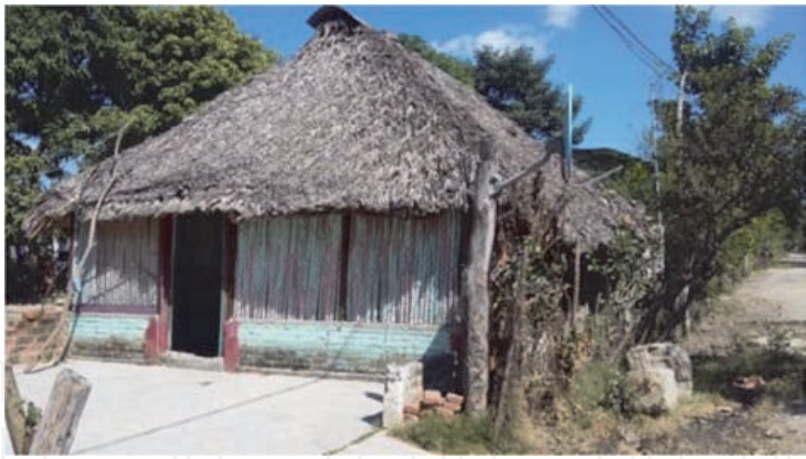
Figure 12. Housing; cane walls and palm roof.
