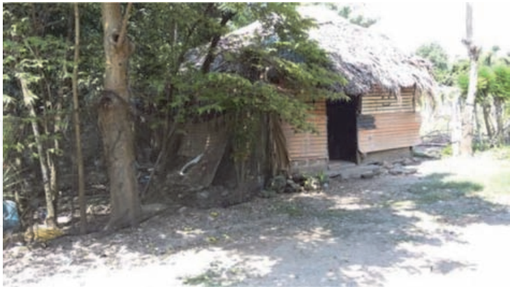
Figure 11. Housing; foil walls and palm roof.
