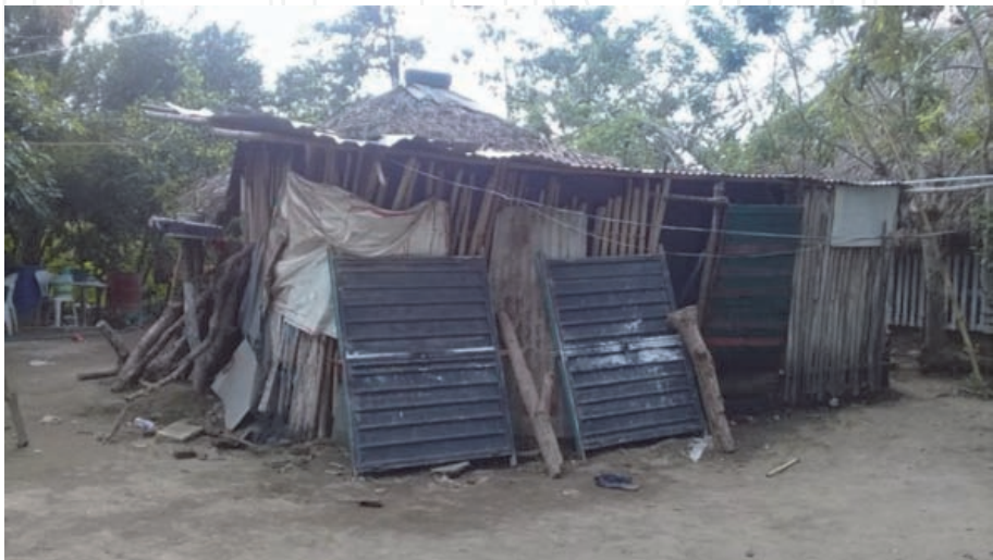
Figure 8. Wooden walls and palm-sheet cover.
