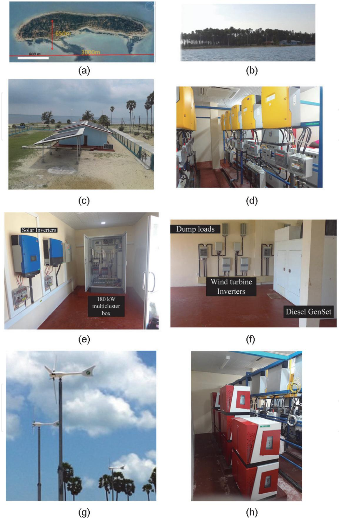
**Figure 14.** Some photos from Eluvithive microgrid. (a) Map of the island, (b) distance view of the island, (c) solar panel and microgrid assembly, (d) solar inverters, (e) solar inverters and multi-cluster panel, (f) diesel generator, wind turbine inverters and dump loads, (g) wind turbines, and (h) Li-ion batteries.
