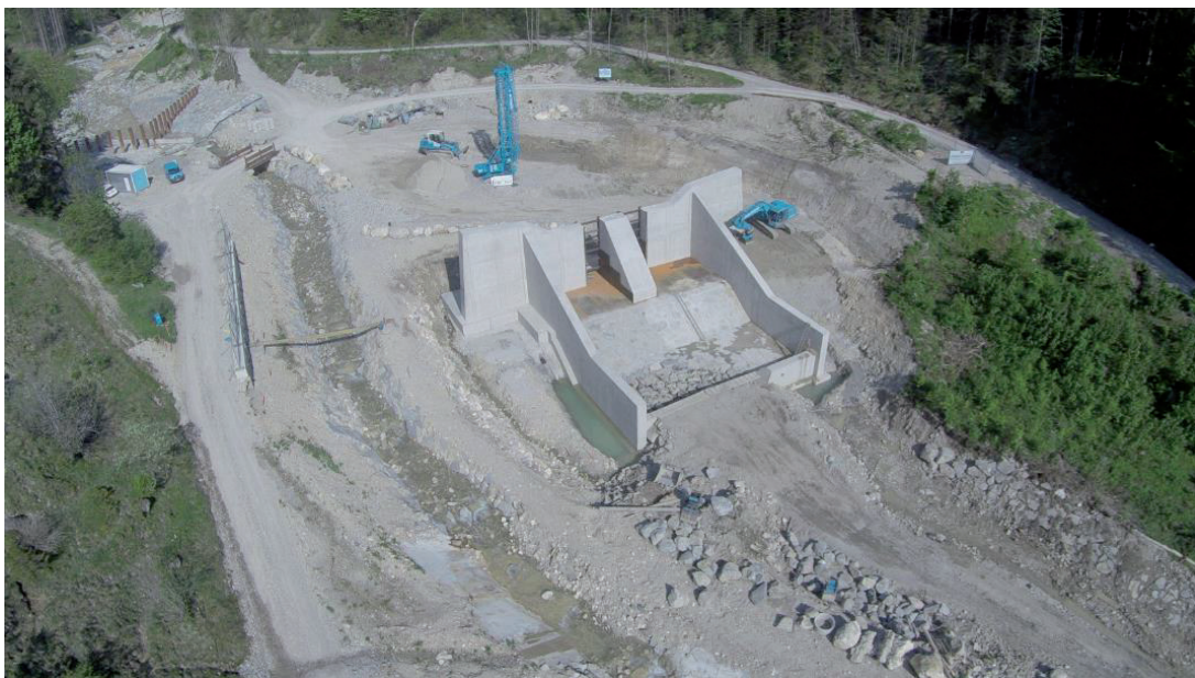
Figure 9. View of the completed barrier structure. A driftwood rake can be seen in the background on the left [12].
