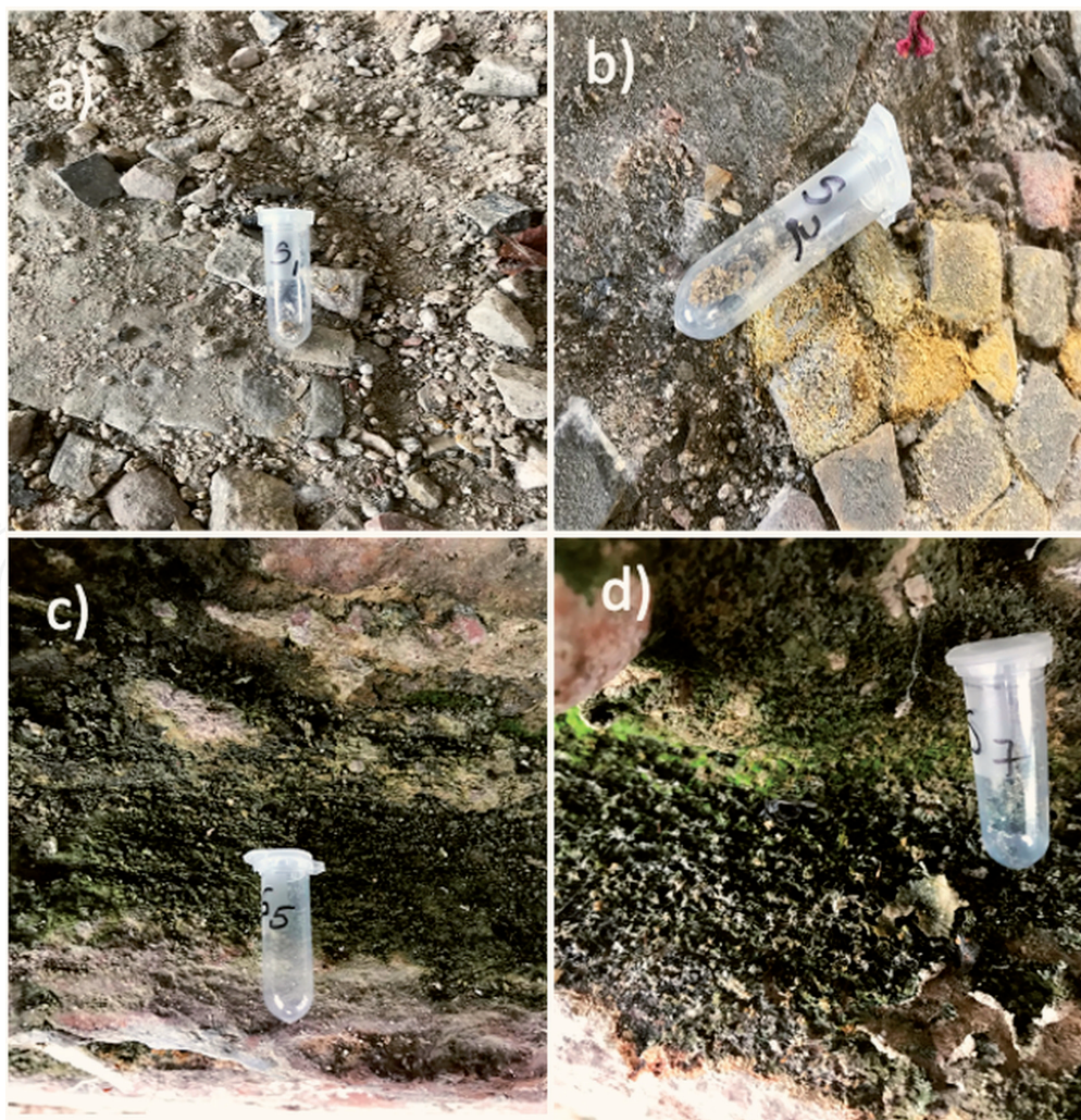
Figure 4. The affected areas of the mosaic by chromatic alteration and destructions (a, b), the biodegradation of wall surfaces (c, d).
