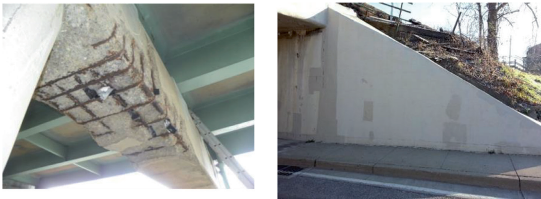
Figure 3. Degradation and retrofitting of highway bridges in West Virginia. (a) Spalling of concrete and exposed rebars of bridge superstructures (courtesy of WVDOT–WVDOH); (b) retrofitting of highway bridge wing walls using GFRP wraps (courtesy of WVDOT–WVDOH).
