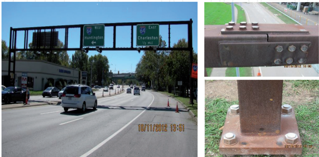
Figure 5. Dual-shoulder-mount-truss weathering-steel overhead sign structures.
