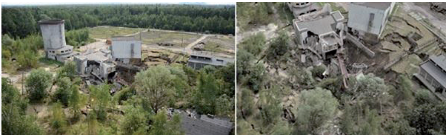
Figure 1. Sinkhole and remains of shaft V, Szczygłowie colliery [6].
