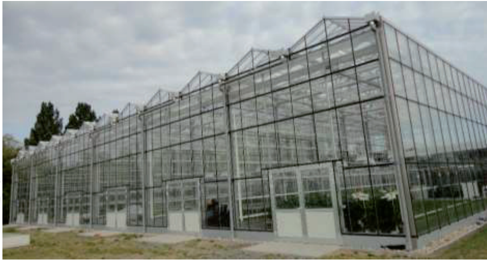
Figure 1. Multi-span Venlo glass greenhouse in Hannover, Germany.
