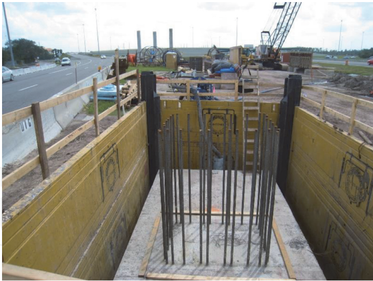
Figure 3. Bridge footing for monitoring in Orlando, Florida.
