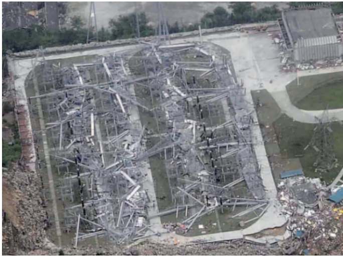
Figure 4. Damage to equipment in the Ertai Shan switchyard.
