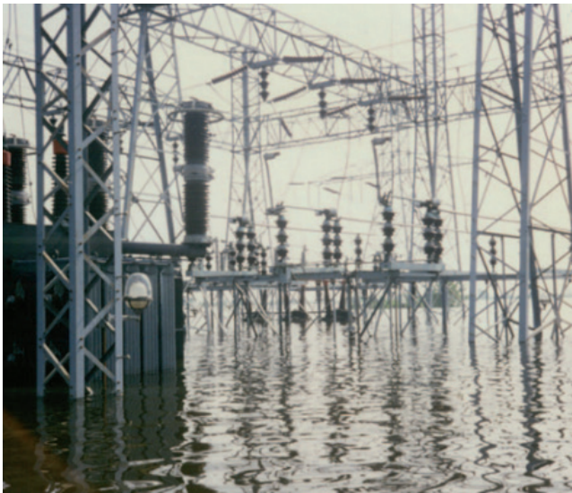
Figure 1. Flooded substations during the 1993 flood at UE.
