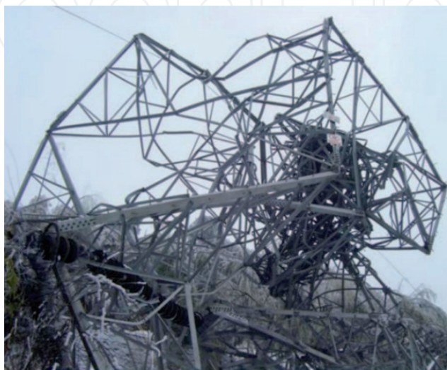
Figure 3. Transmission tower collapse caused by ice accumulation.
