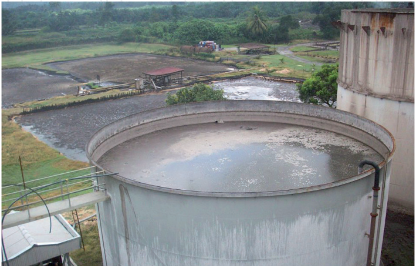
Figure 5. Typical open digester tank.
