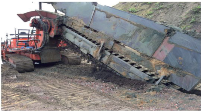
Figure 16. Installation of the deep drainage.
