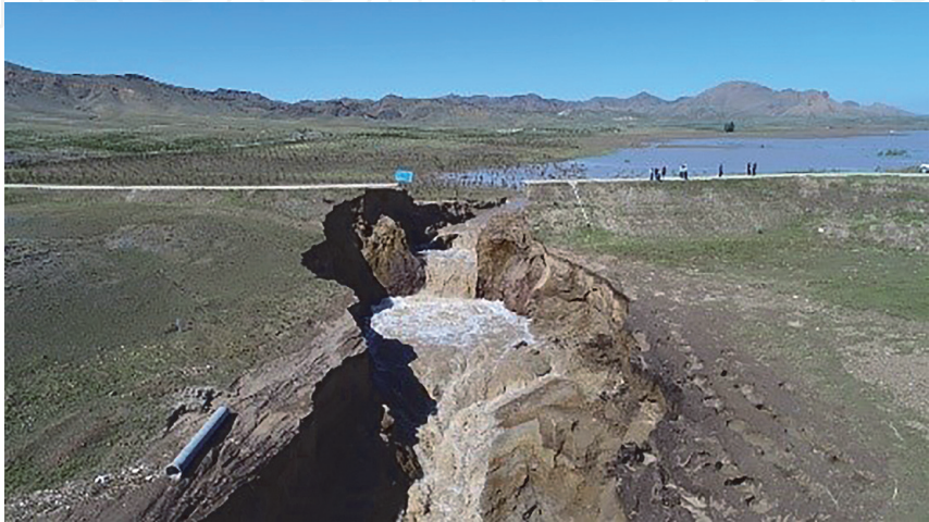
Figure 3. Final breach of Zenglongchang dam.
