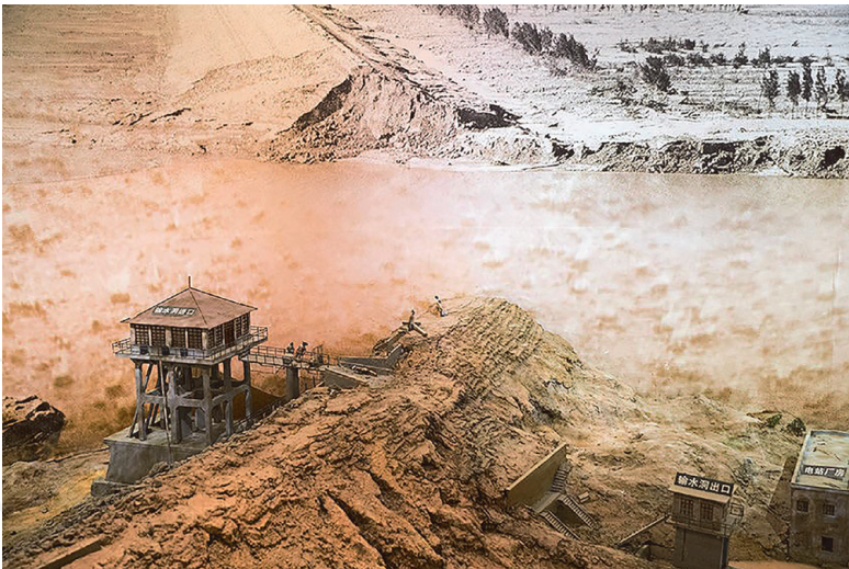
Figure 1. Final breach of Banqiao dam.
