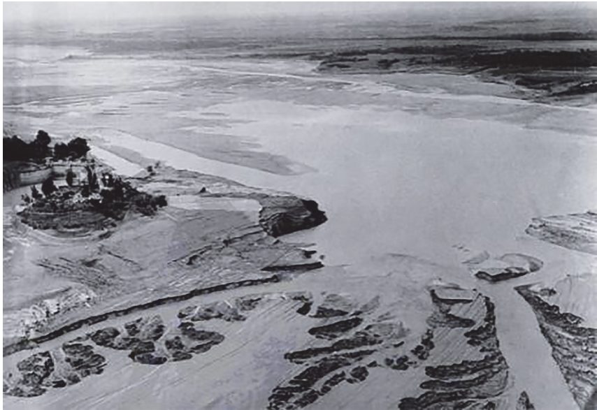
Figure 2. Final breach of Shimantan dam.
