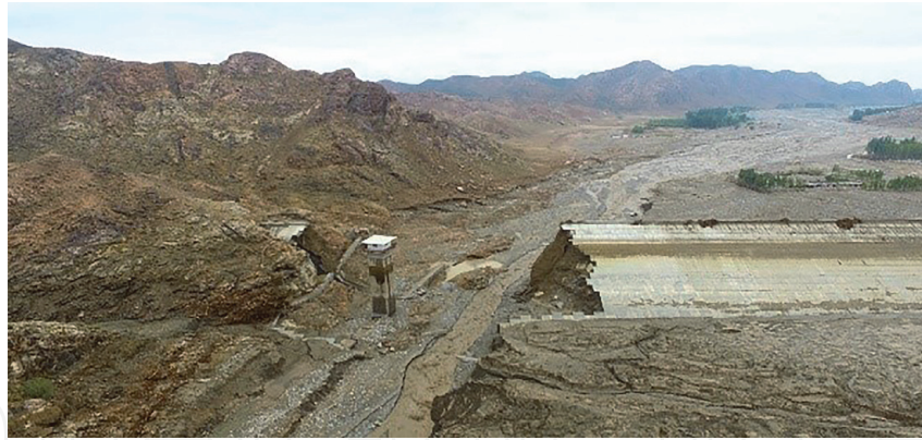
Figure 4. Final breach of Sheyuegou dam.
