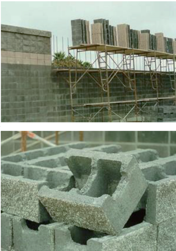
Figure 3. Brick and masonry noise barriers.
