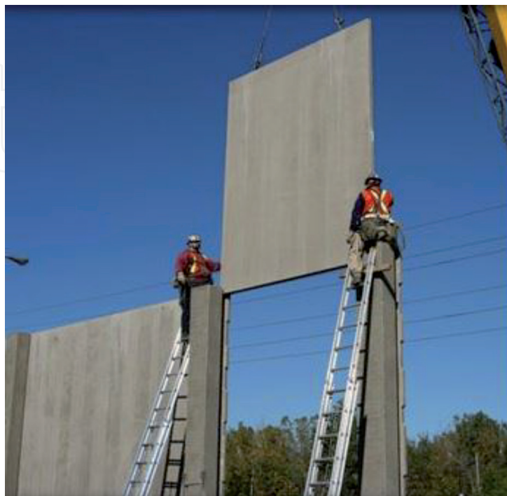
Figure 5. Precast concrete noise barriers.
