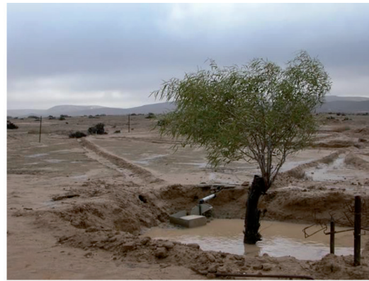
Figure 6. Traditionally designed micro-catchment system: (a) schematic of the system and (b) flooded micro-catchment.
