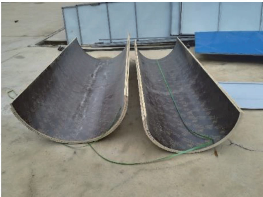
Figure 4. Molds for concrete casting.
