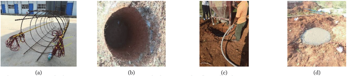
Figure 9. Construction steps of cast-in-place ordinary concrete piers for foundation casting. (a) Prepare reinforcement; (b) manually dig the hole; (c) put the steel cage into the hole, followed by concrete casting and consolidation; (d) seal the top with membrane to prevent evaporation of water.
