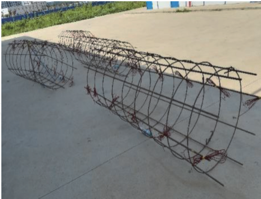
Figure 3. Steel reinforcement cage.
