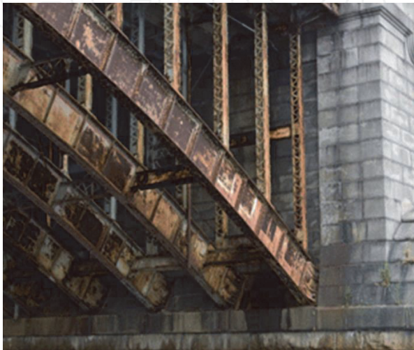
Figure 20. Bridge of structural steel with corrosion problems [19].
