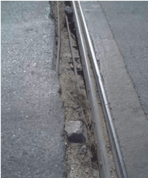
Figure 21. Bridge concrete construction joint damaged [20].
