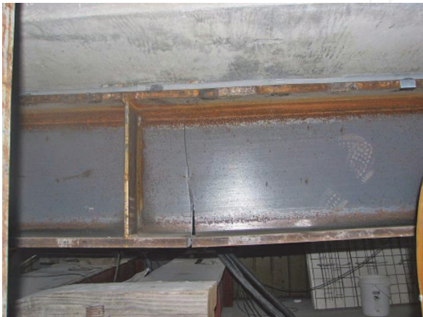
Figure 22. Steel beam with fatigue crack failure [21].
