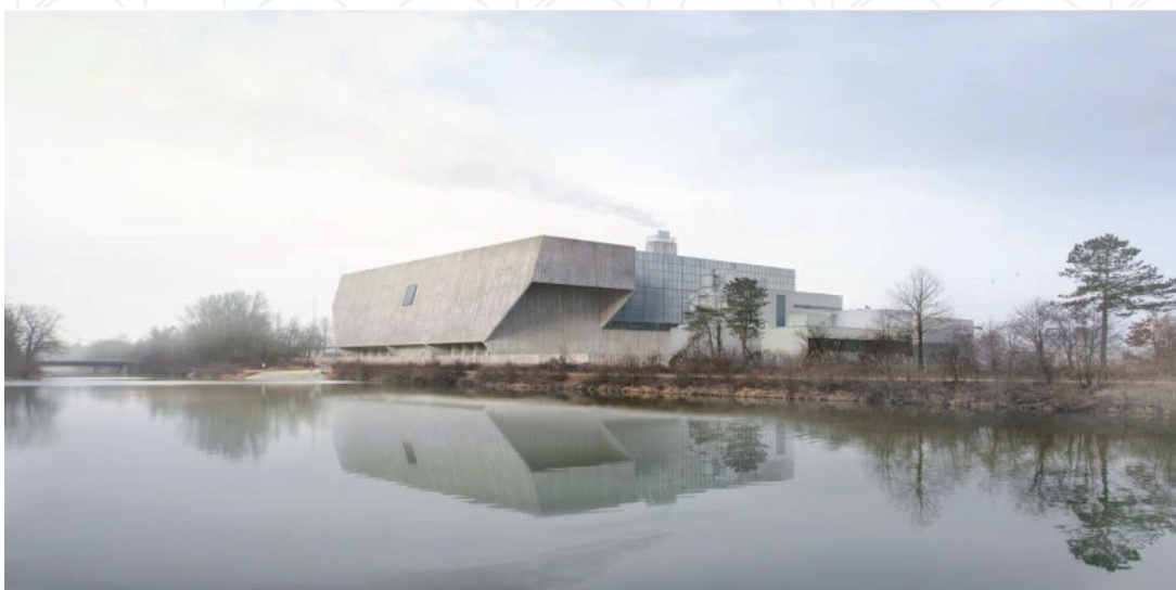
Figure 9. KVA Thun energy-from-waste plant of 100,000 tons/year of combustible waste with energy recovery: electric power about 12 MW (maximum) and district heating output about 25 MW (maximum) [23].
