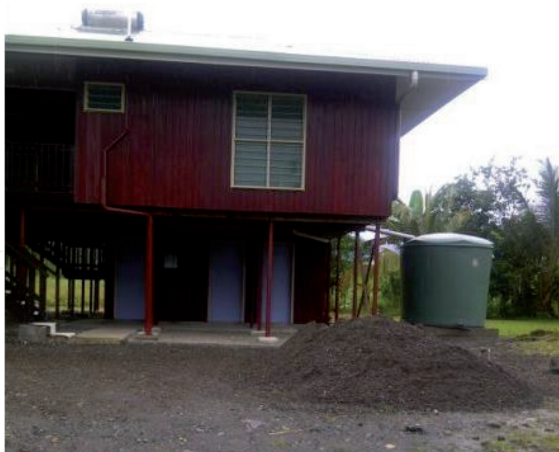
Figure 3. Rainwater harvesting system (RWHS) via rooftop at Papua New Guinea University of Technology. (Adapted from Betasolo and Smith, 2017.)
