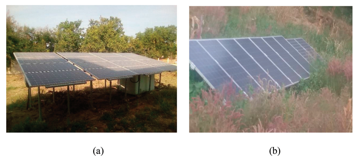
Figure 5. (a) Soiling and dust accumulation and (b) vegetation.
