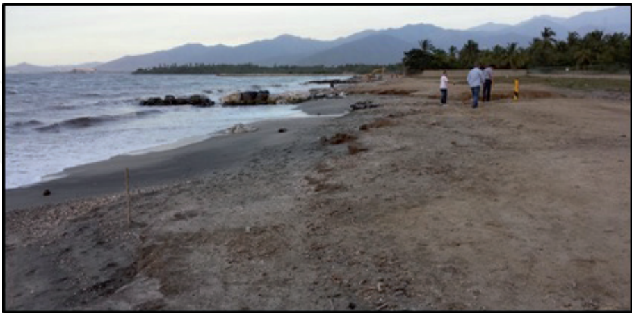
Figure 21. Severe beach erosion along the Costa Verde Cienega coast, exposing a crucial pipeline (yellow marker). Note the low-profile sandbag groin and the earth-moving machine at the top of the picture. The earth-moving machine was moving sand from the upland to nourish the beach and attempting to control the erosion.
