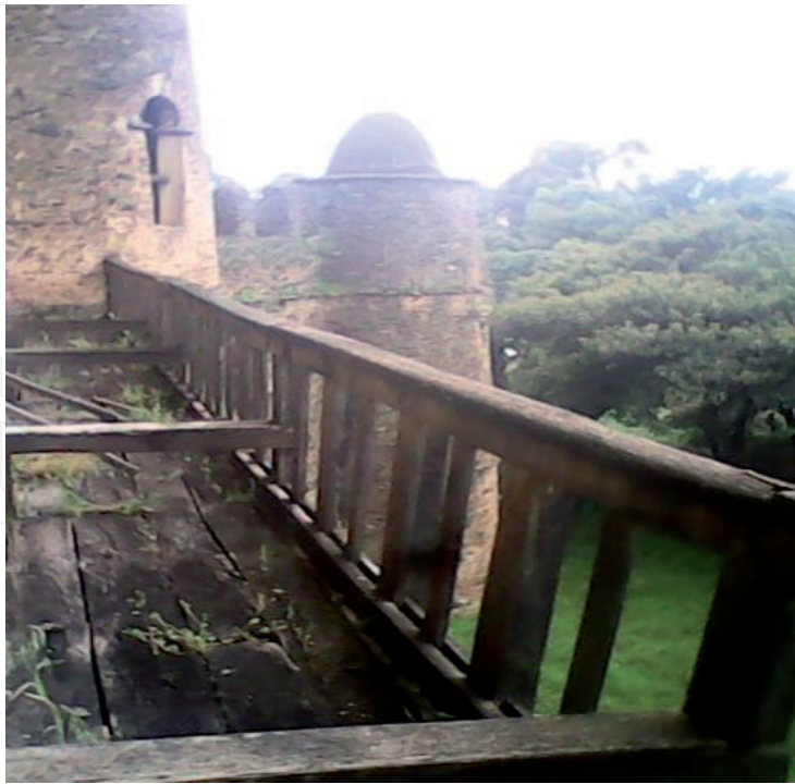
Figure 6. Active durability issue due to the presence of grass and alga on the wood floor terrace [source; Eskinder Desta].
