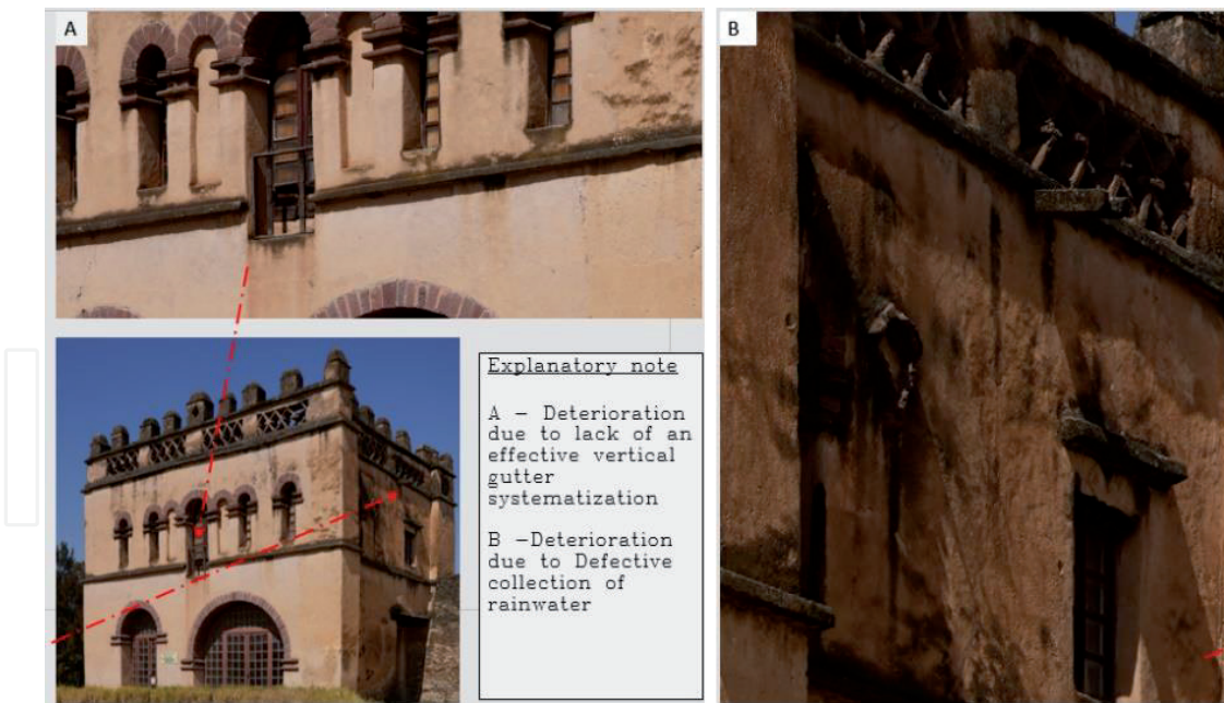
Figure 2. The effect of improper rainwater removal on the face of the wall [29].
