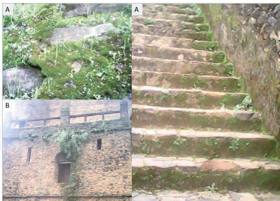
Figure 3. The progressive biodeterioration processes on the surface of building materials: algae constitute the medium for the growth of fungi that pass through the building material by means of their hyphae. Dense formations of herbaceous plants [A] vascular plants [B] mosses and algae [source; Eskinder Desta].
