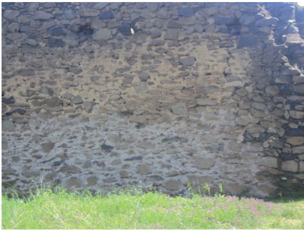
Figure 4. A widespread lack of binding mortar in between the stone masonry [source; Eskinder Desta].
