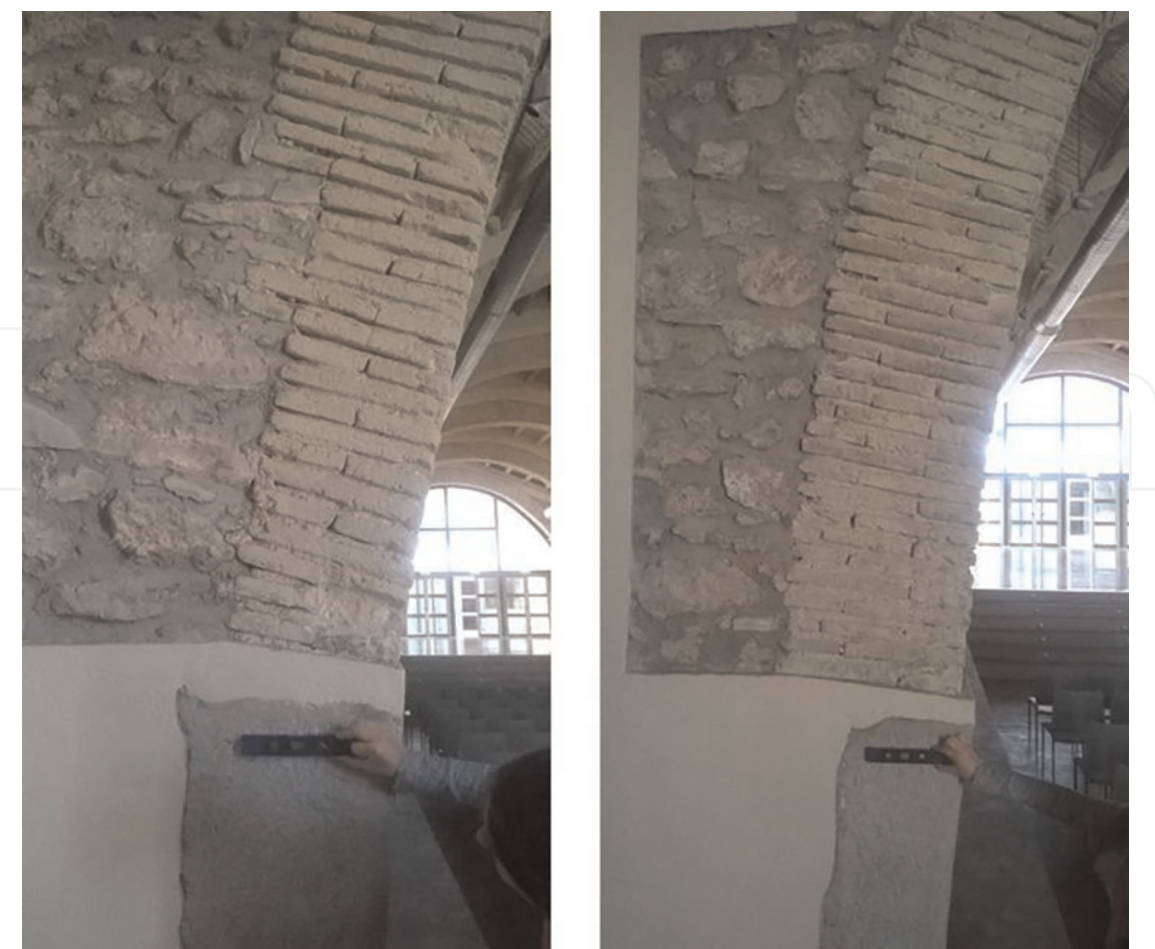
Figure 21. Springing of arches no. 1 and no. 2 in the O'Connor cellar.
