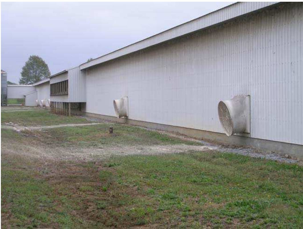
Fig. 6. Fan Arrangement on lower story of hen house. Small extension of building near background has a set of six fans protected to reduce light entry into the building.
