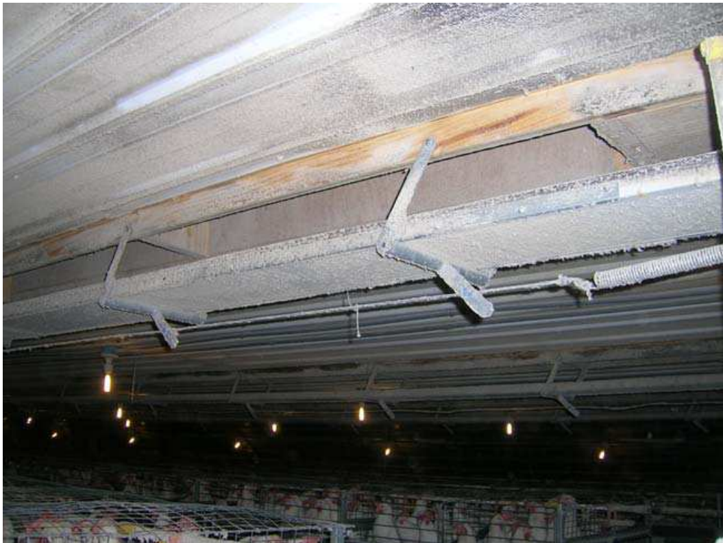
Fig. 5. Horizontal baffle with inlet slot above it is adjustable to match inlet area to air flow capacity of operating fans.
