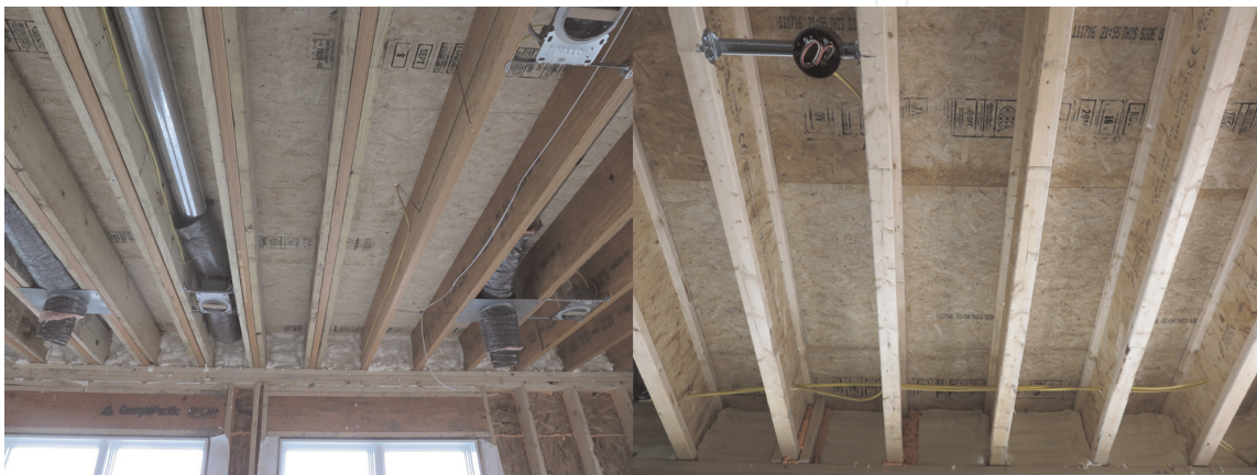
Figure 4. Typical I-joist and LVL (courtesy Timber Rock Homes).
