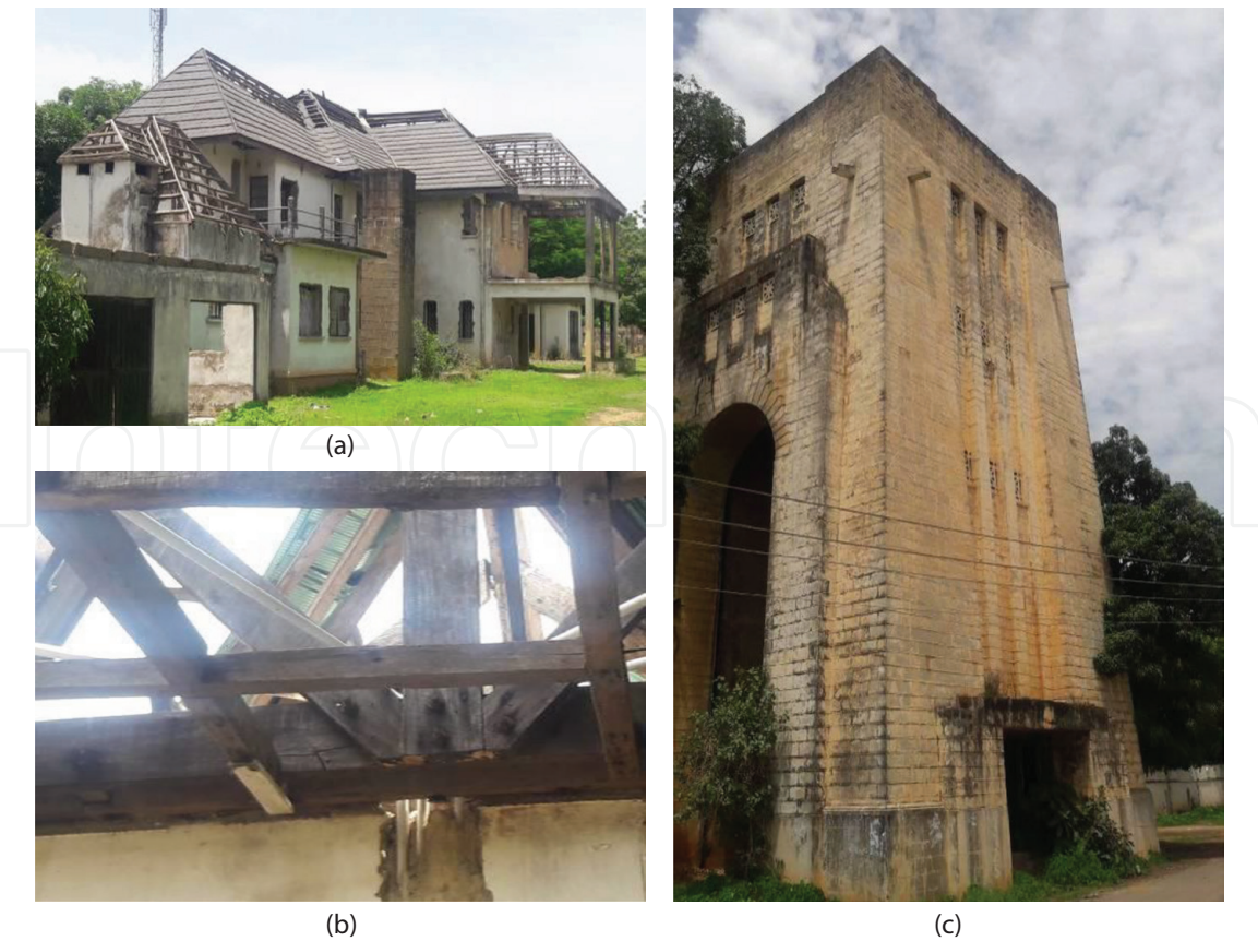
Figure 4. (a and b) Lord Frederick Lugard residence as you approach and the roof trusses showing well-seasoned timber bolted and secured for about a century. (c) Lord Frederick Lugard residence Water Tower often used as a watch tower during early days of Kaduna township development.
