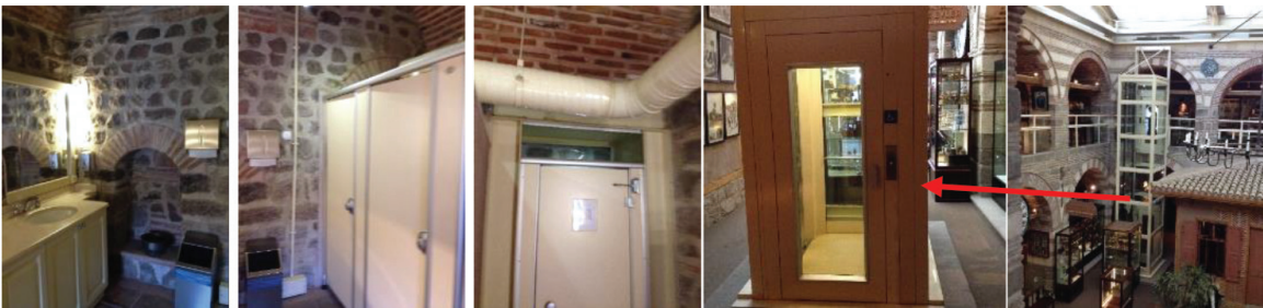
Figure 7. Interior additions in Çengel Khan are mostly observable at mechanical installations, handicapped lift, and door and window alterations and at designing wet spaces [39].
