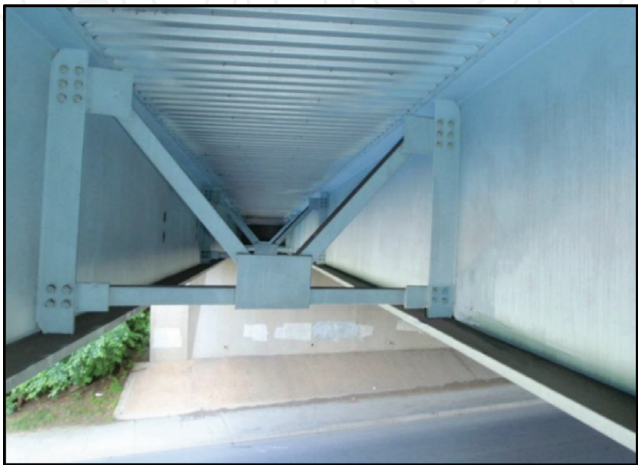
Figure 4. K-type cross brace on Middlebrook Bridge.
