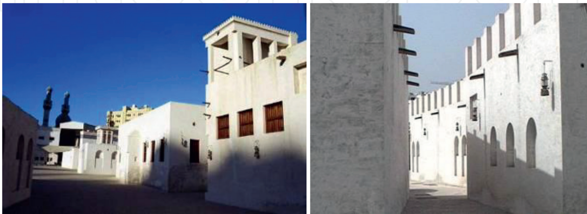
Figure 3. Accommodation to the ambient environment in vernacular architecture in the Arab World: solid walls, small openings, light finishing, courtyards, and wind catchers (Source: Salman, Maha).
