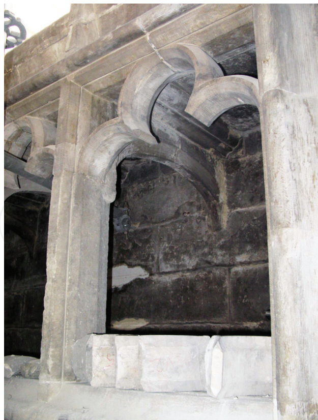
Figure 2. Repaired tracery with damaged elements in Notre Dame du Sablon (photo by M. Drdácý).
