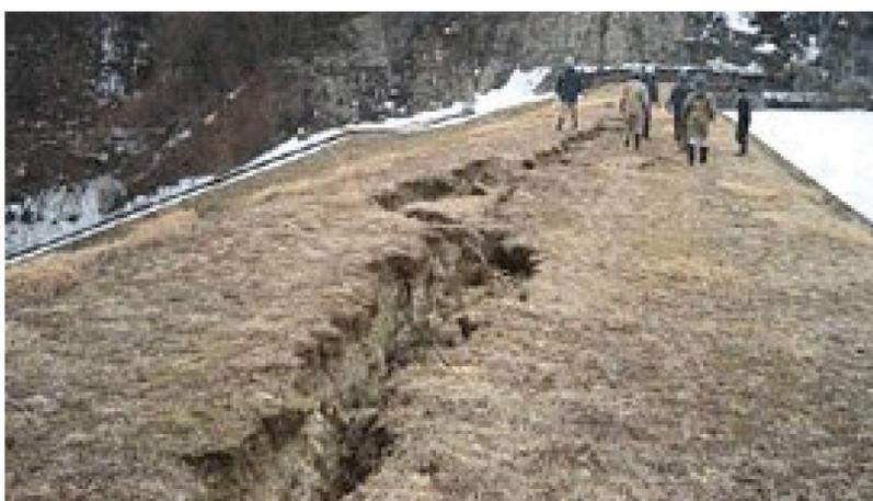
**Figure 1.** Crack at the Earth-fill dam.
