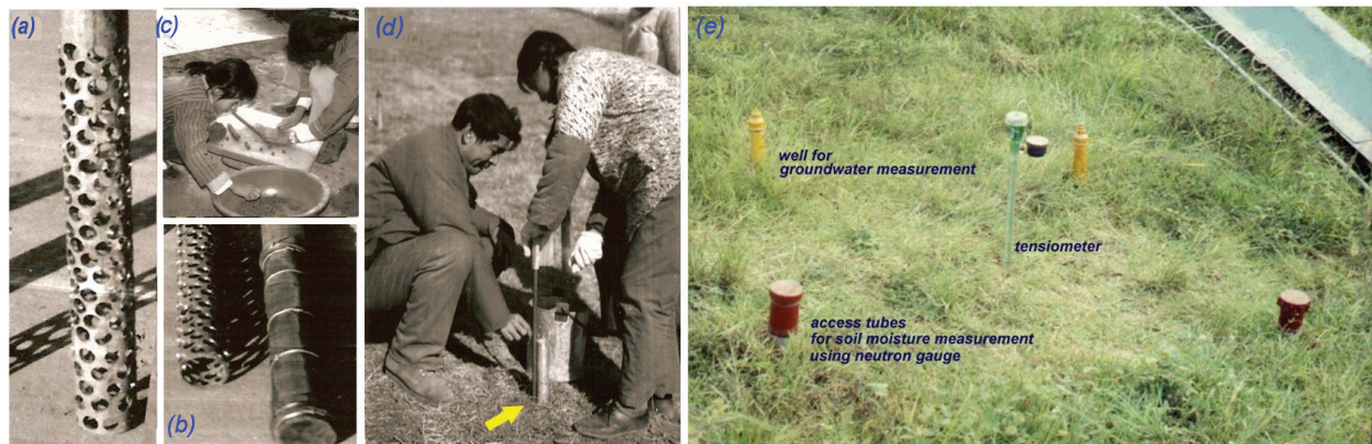
Figure 10. Construction of groundwater monitoring well. (a) the slotted part of steel tube; (b) the tube was wrapped up by plastic net; (c) making clay balls for using; (d) during installing, the space between the tube and drilling hole above the slotted lengths (shown by a yellow arrow) should be carefully stuffed up by small dried clay balls using a special designed tool. This picture is shown in commemoration of the late prof. M-Q Lu (left) of Nanjing University for his efforts and contributions. (e) a part of resulted networks showing well for groundwater, access tube for neutron moisture measurement using neutron gauge and the tensiometer with connection plastic tubes to the scanner.
