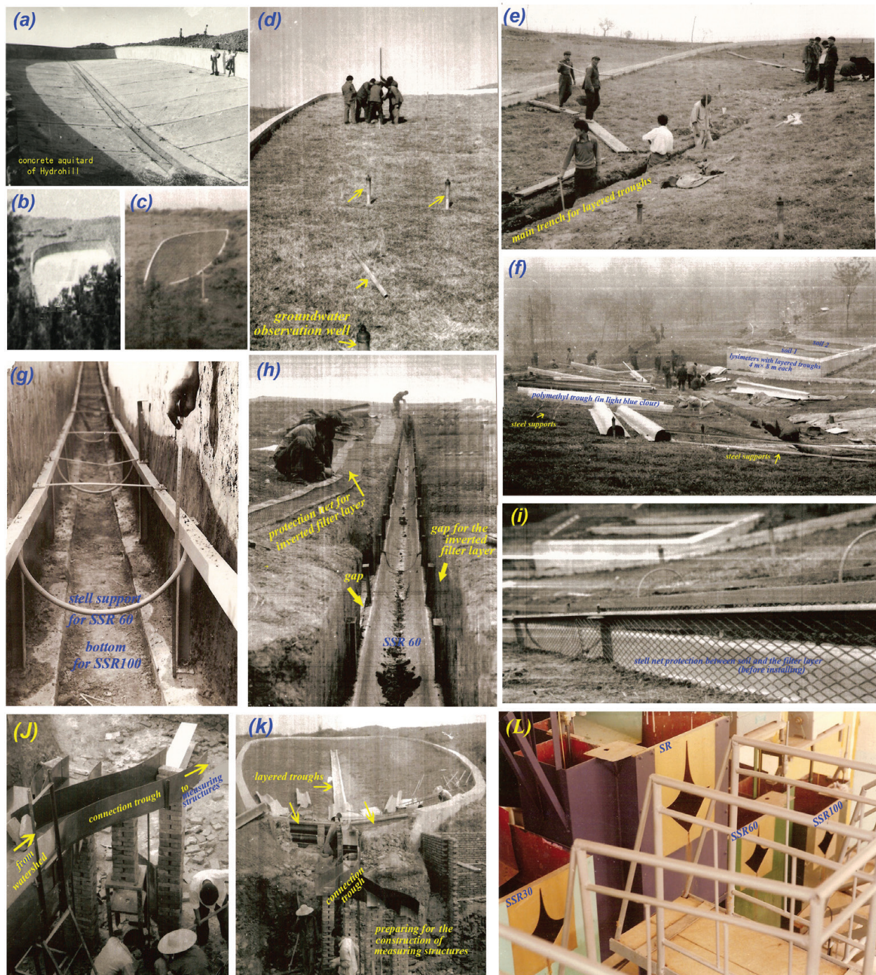
Figure 9. Constructions of Hydrohill. (a) the artificial aquiclude and surrounding wall; (b) view of the completed concrete aquiclude and wall; (c) view of the artificial catchment while soil was filled up, it was in idle for 3 years waiting for the physical improving of filling soil; (d) setting up monitoring networks for both saturated and unsaturated zone; (e) set drainage trenches; (f) the splicing fiberglass troughs and some steel supports; (g) the rectangular bottom trough for SSR100 and steel supports for the setting of SSR60 trough above it; (h) the gap for inverted filter and the nylon net in preparing; (i) the stainless steel screen in preparation for setting; (j) a curved connection trough; (k) connection troughs in installing; (l) discharge measuring structures using V-notch based logarithm sharp crested weirs (1982–1995).
