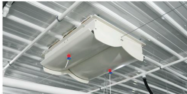
Figure 4. Example ceiling fresh-air diffuser commonly used in HLPP systems. The cable shown passing through the diffuser is used to automatically control baffle opening in response to ventilation rate changes with static pressure control as the ultimate diffuser opening control objective.
