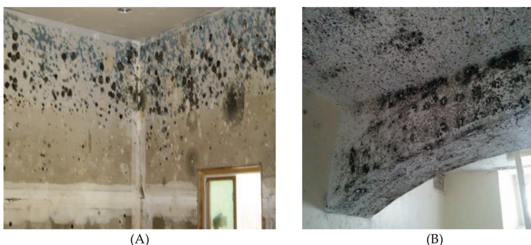
Plate 3. (A) Damped roof in a building in Bere Area of Ibadan, and (B) mould growth on wall and ceiling of a typical house in Ibadan.
