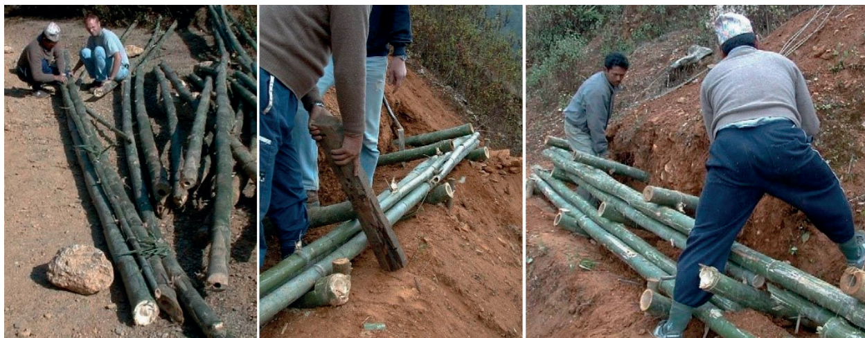
Figure 1. Crib wall construction steps in Thankot (Nepal) 2002 [7].
