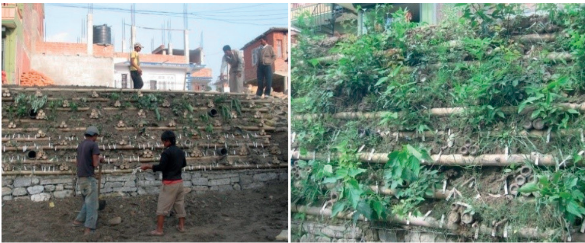
Figure 7. The vegetated bamboo crib wall just after construction (November 2006) and after 1 year of construction (Kusunti, Lalitpur, November 2007) [26].
