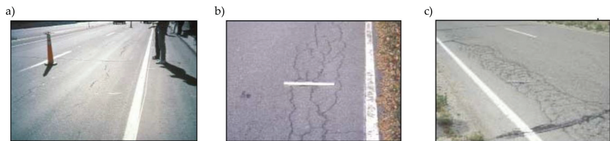
Figure 5. Fatigue failure of asphalt concrete pavement for the highway according to the Guide [13]: (a) low level; (b) middle level and (c) high level.
