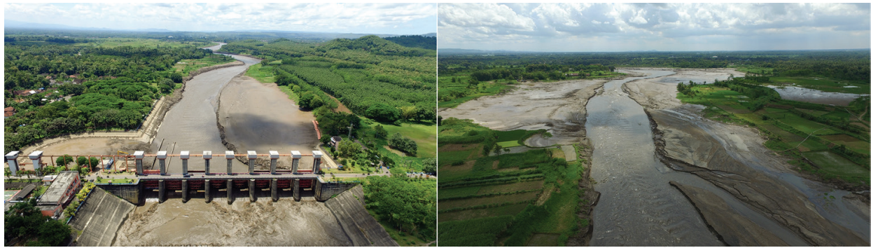
Figure 5. Aerial views of Wlingi (left) and Lodooyo (right) reservoirs taken by a drone showing sediment deposition in the reservoirs during sediment flushing on 25–26 March 2016.
