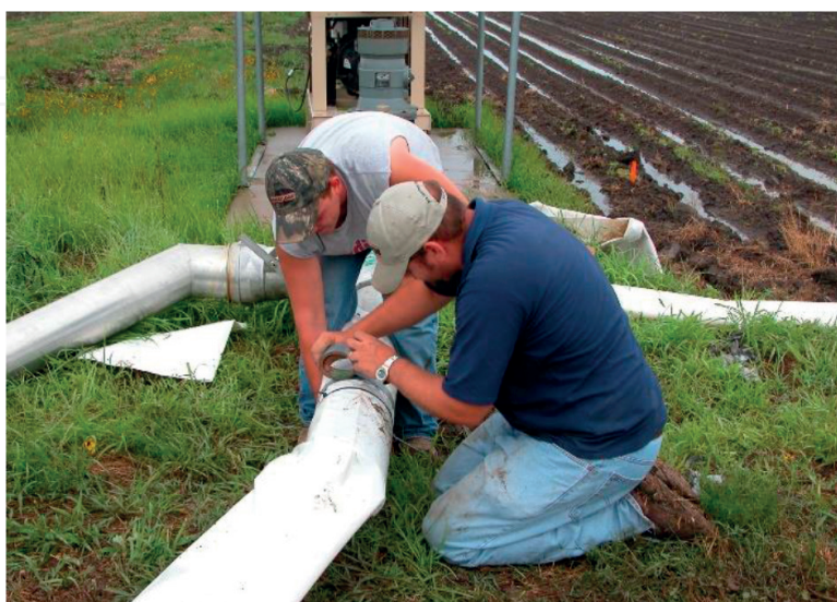
Figure 2. Connecting plastic tubing to well pipe with zip ties and duct tape.
