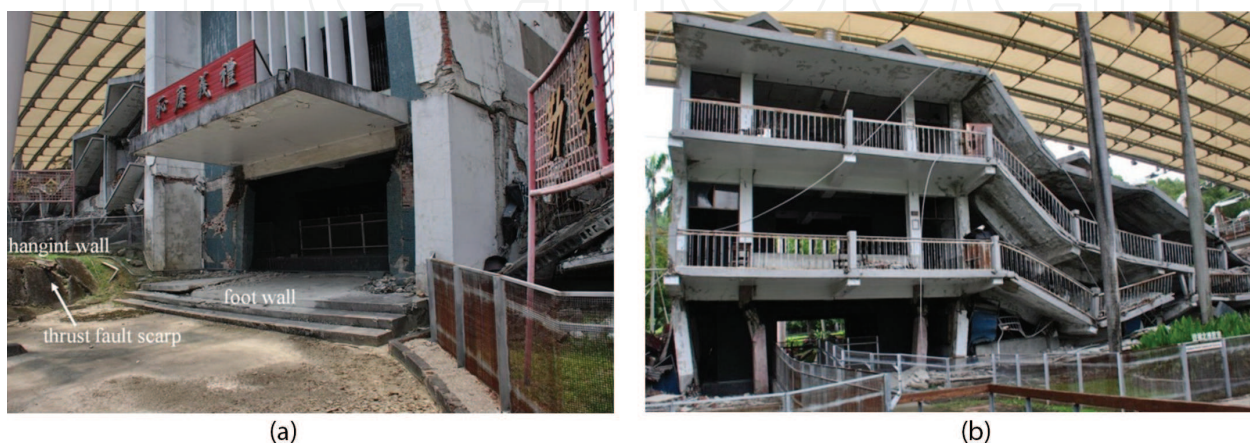
Figure 7. The collapse of the Kuangfu junior high school building during the Jiji earthquake: (a) front view; (b) rear view.
