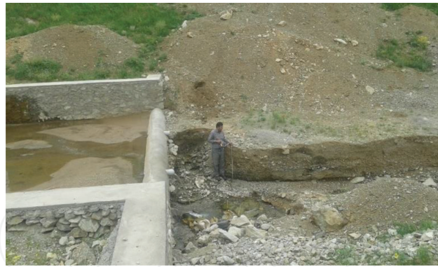
Figure 2. Misconducting of a check dam on a water way.
