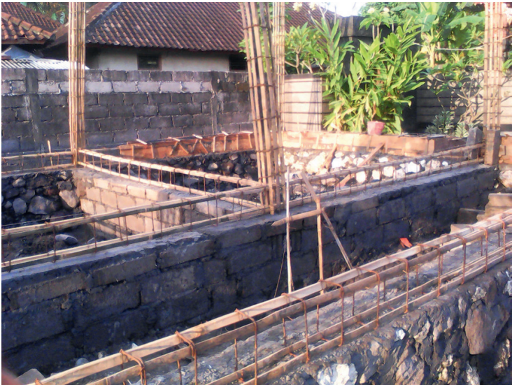
Figure 9. The bamboo reinforcement was assembled before concrete was casted [24].
