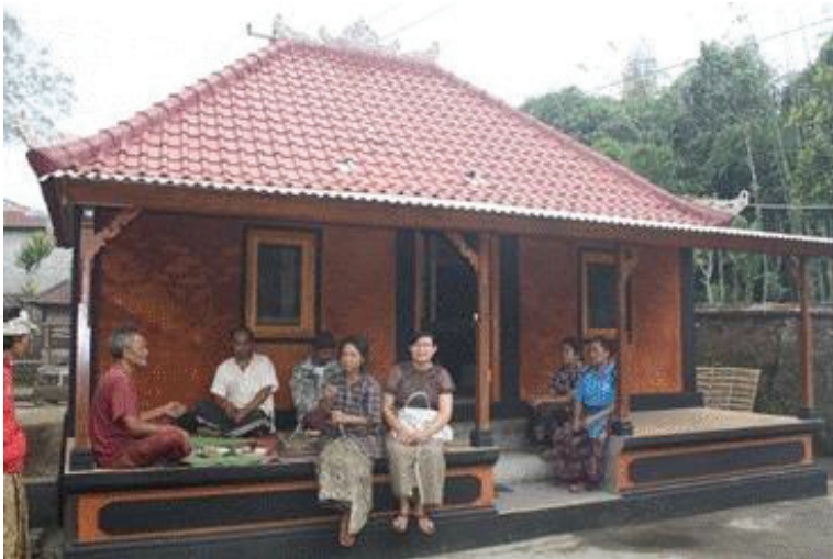
Figure 10. The simple traditional Bali age house with the bamboo reinforced concrete structure and brick walls [23].
