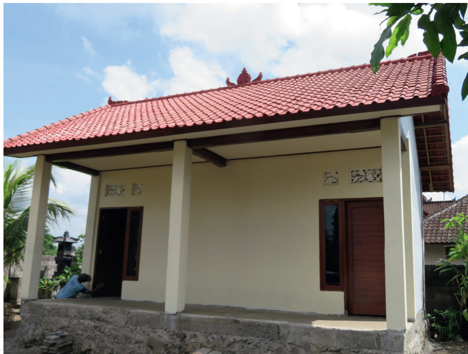
Figure 12. The simple modern Balinese house with the bamboo reinforced concrete structure and concrete block wall [24].
