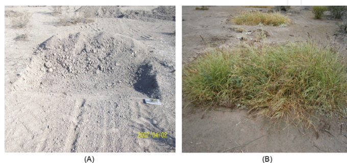
Figure 5. Micro-watershed for water harvesting; when was built (A), and after, when the grass has grown (B).
