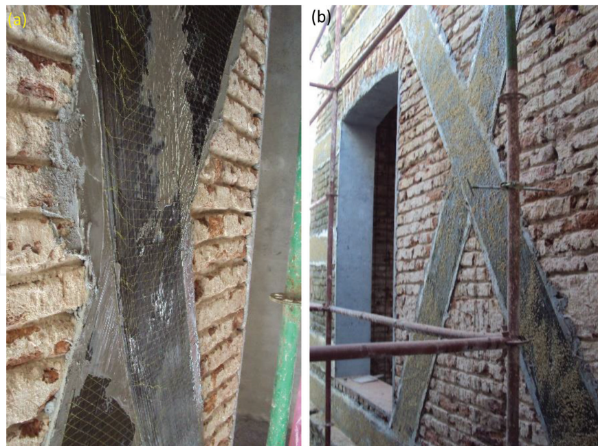
Figure 4. Carbon fiber wrap applications on masonry walls (a and b).
