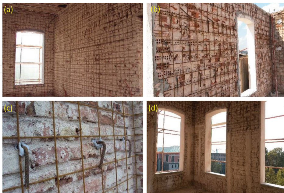
Figure 5. Retrofitting of the internal walls after plaster removal: (a–c) rebar grid technique and (d) application of thick plaster.
