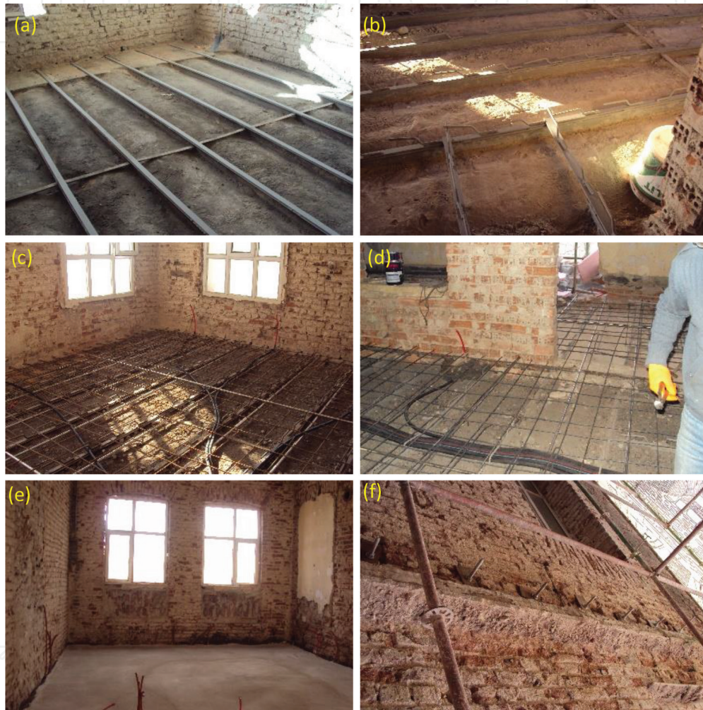
Figure 6. Retrofitting of jack arched slabs: (a) removing top layers of the slab, (b) welding of shear rebar over I-profile beam, (c) steel tie, (d) connections of stainless steel ties between the masonry walls, (e) anchorage of stainless steel, and (f) topping concrete application on slab.
