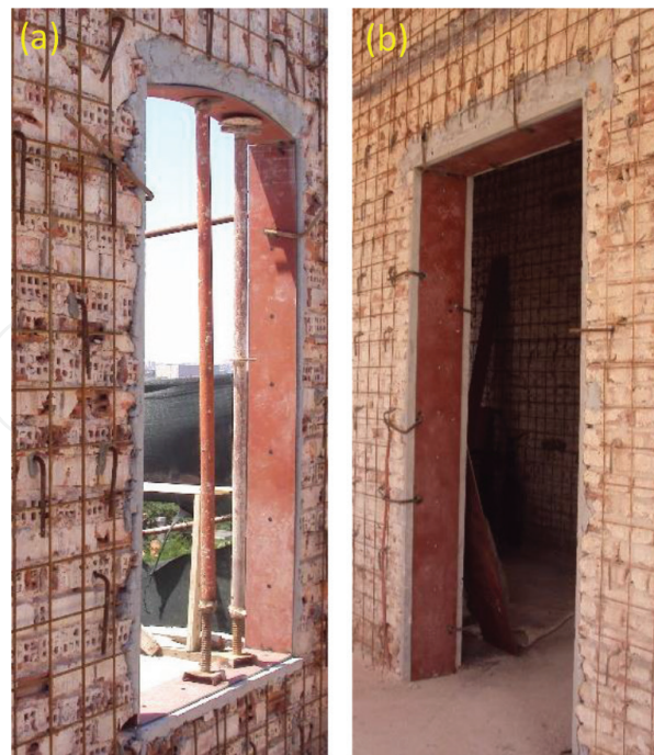
Figure 7. Retrofitting of door and window gaps using steel plates (a and b).
