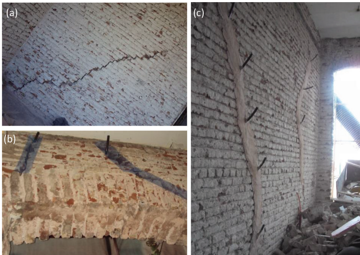
Figure 3. Injection application in the walls after plaster removal: (a) structural cracks, (b) preparation of wall surface for injection, and (c) injection application by manual technique.
