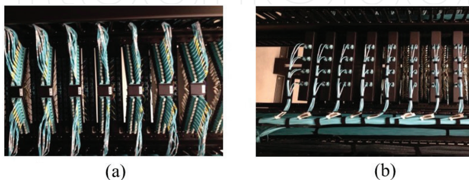
Figure 2. Example of optical fiber wiring (a) with single-fiber connectors and (b) with multifiber connectors.
